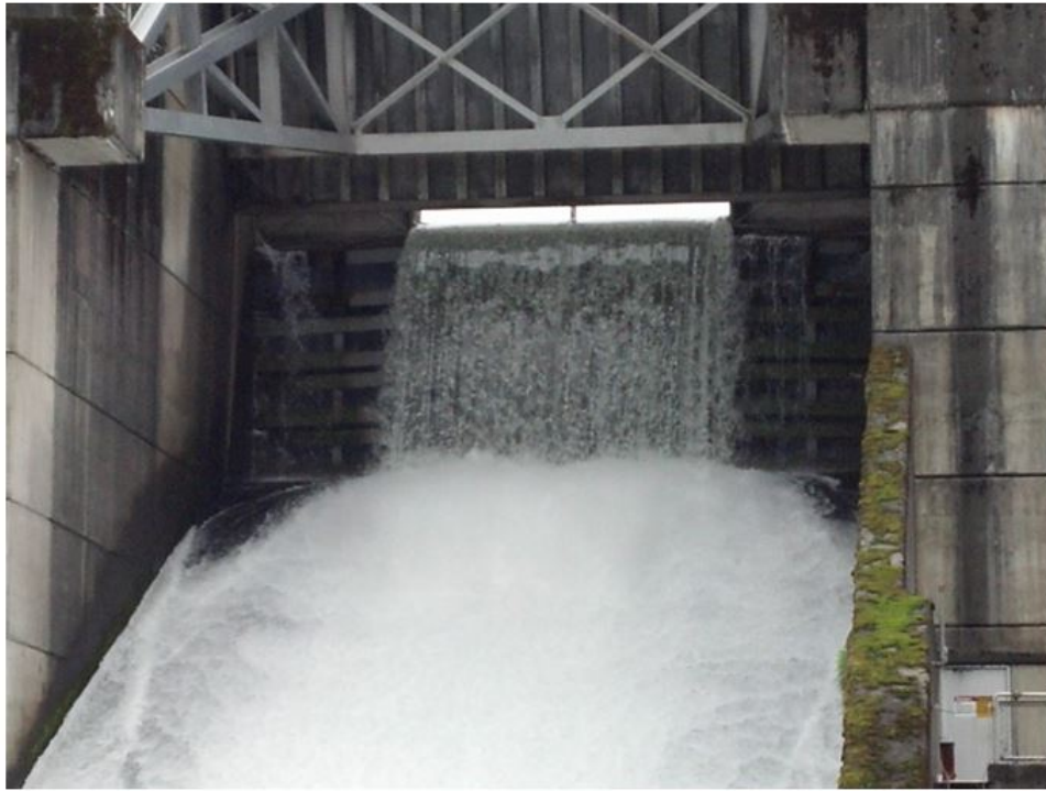
Figure 3-4 – Top: CFD of Existing Weir at Approximately 200 cfs; Bottom: Existing Weir at Approximately 200 cfs
