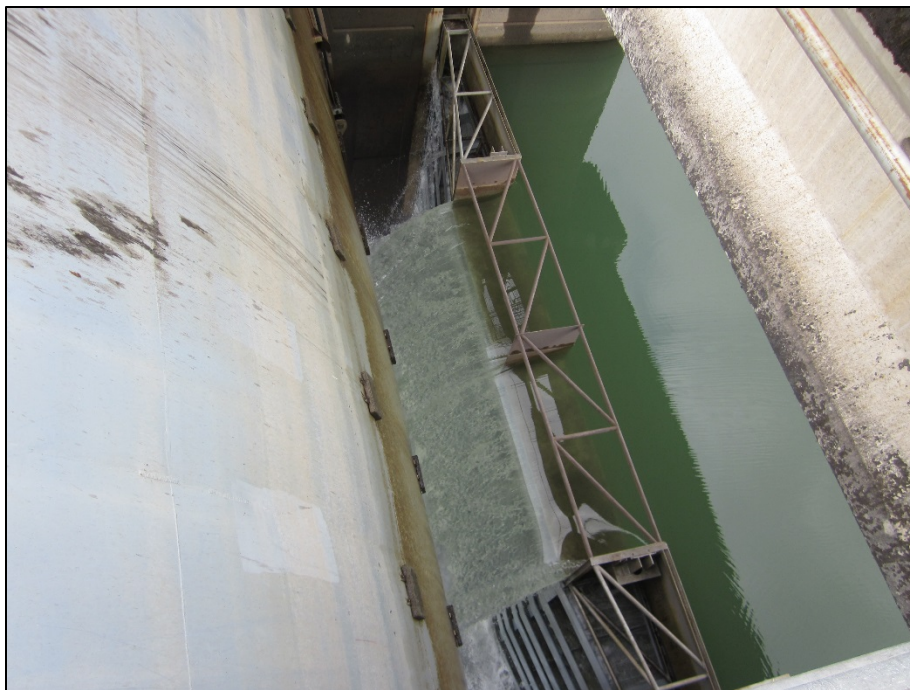
Figure 4-1: Existing Foster Dam spillway passage fish weir during operation.
